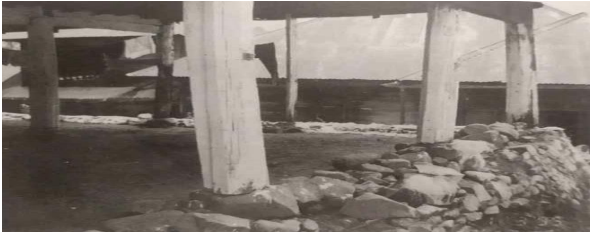
Figure 9. A single slab stone as a pillar foundation
