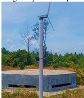
**Gambar 3.** Turbin angin sumbu horizontal
